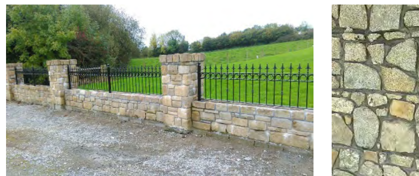
Example of Granite Wall and Railing similar to that proposed at the Brennanstown Road boundary.
