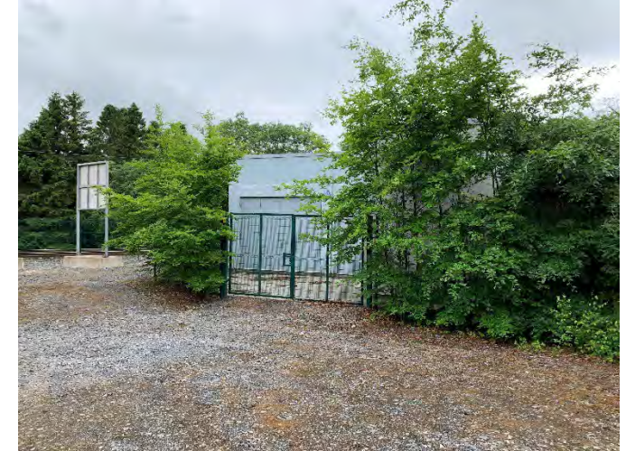
V7 - Luas Substation in south of site
